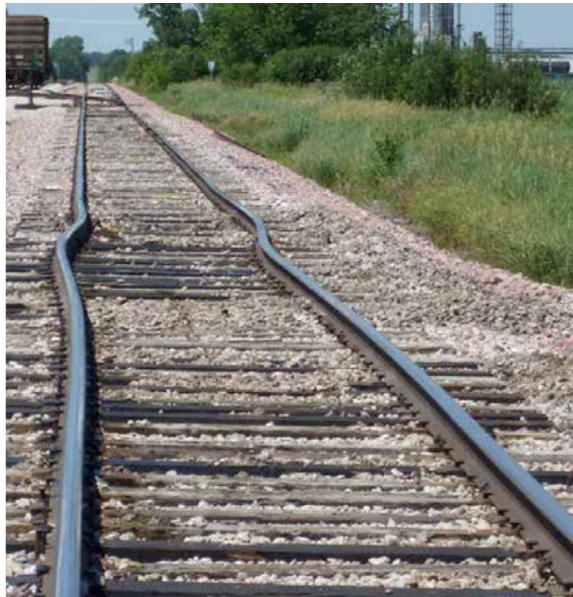
Figure 8.4. High temperatures can lead to rail deformations such as the “sun kinks” seen here on rail lines in Iowa (Photo: Iowa Department of Transportation).
