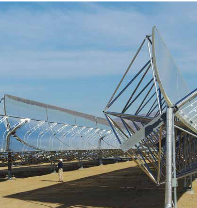
Figure 7.6. Arvada-based SkyFuel designs and builds concentrating solar power (CSP) plants like the parabolic trough plant pictured here in Nevada. Although no utility-scale CSP plants have been built yet in Colorado, they have been proposed and are appealing due to their lack of significant greenhouse gas emissions. The decision of whether to use water versus other substances (like molten salt, as used in this facility) as a heat transfer fluid will determine the level of impact that any new proposed CSP facility would have on water and other sectors (Photo: SkyFuel, http://www.SkyFuel.com ).
