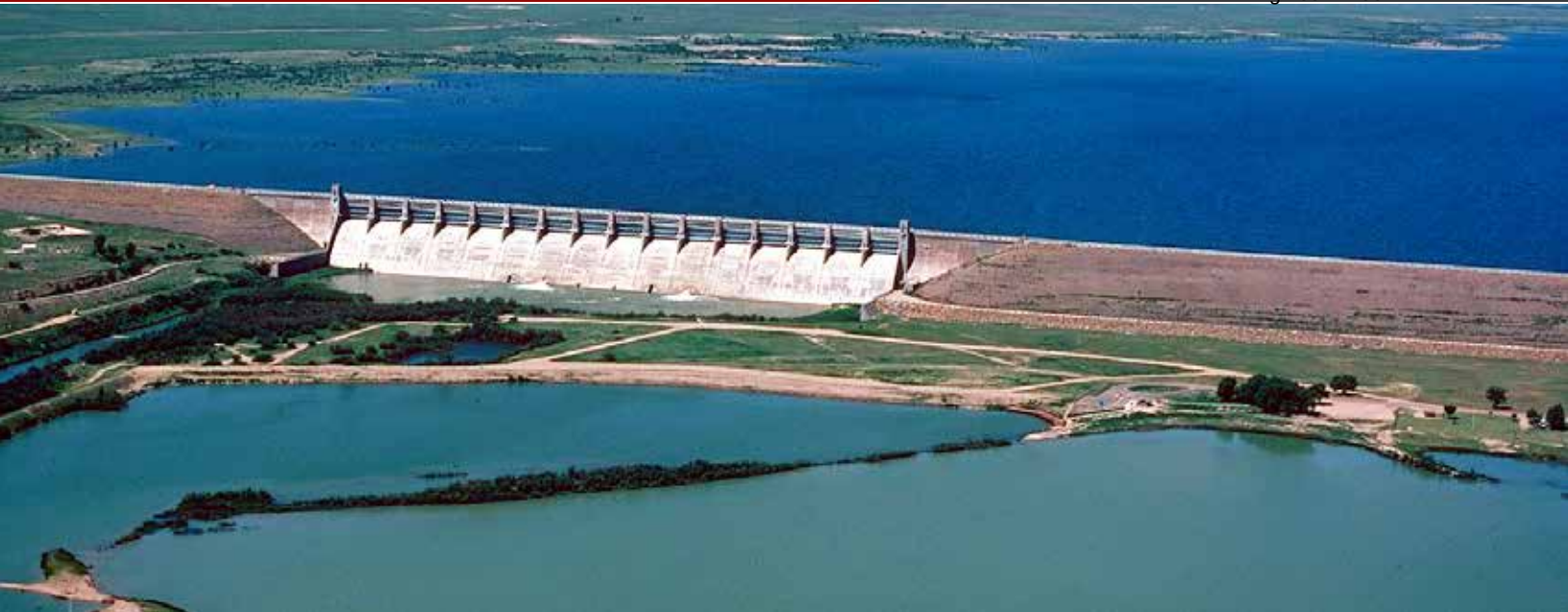
John Martin Dam and Reservoir on the Arkansas River in Bent County, Colorado. Photo: U.S. Army Corps of Engineers Digital Visual Library.
