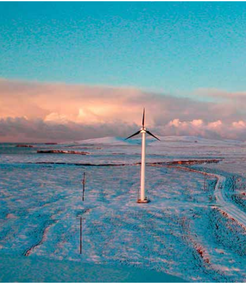
Figure 7.4. Snow and other winter weather conditions can negatively affect wind turbine operations (NorthWind 100 turbine in Toksook Bay, Alaska. Photo: National Renewable Energy Laboratory).
