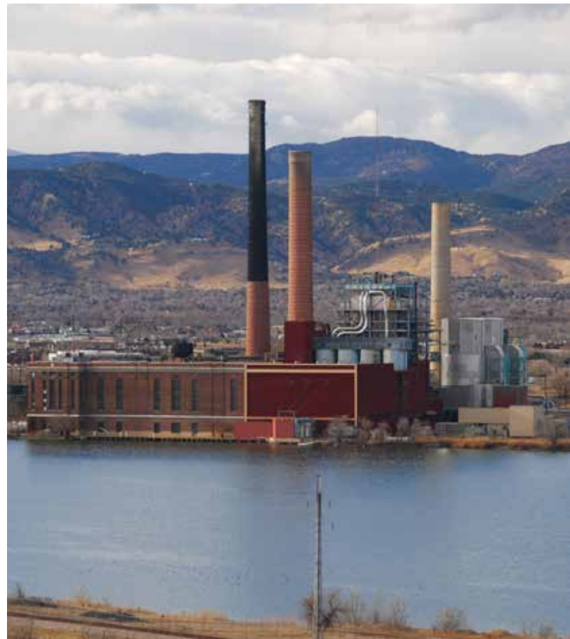
Figure 7.3. Xcel Energy's Valmont Power Plant in Boulder uses water stored in three surrounding reservoirs for cooling (Photo: Creative Commons, Let Ideas Compete).
